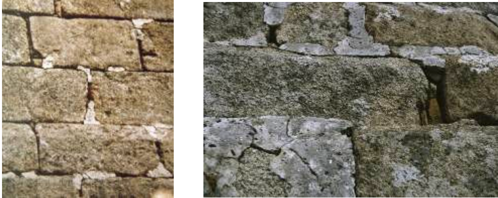
Figure 1. Deterioration process at S. Xiao Moraima due to the use of cement-based mortars
